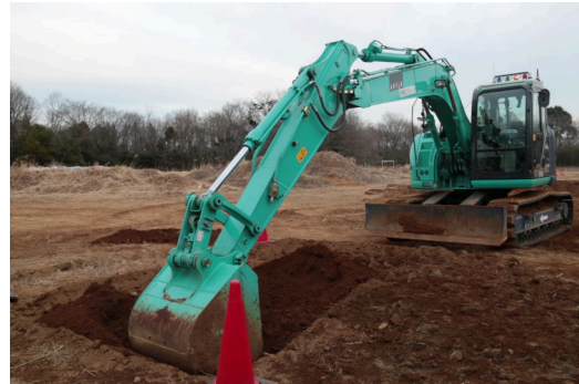
Figure 9: Digging the land and filling
