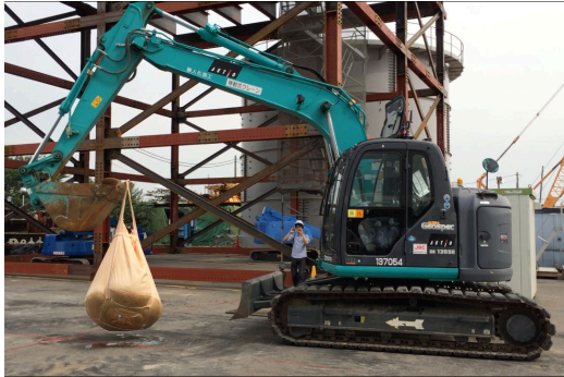
Figure 8: Picking up a Sand Sack and Placing on a Crosshair marked on tarmac
