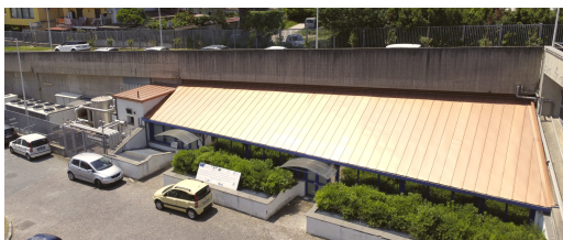
Figure 7: Data Center in the Federico II University of Naples
